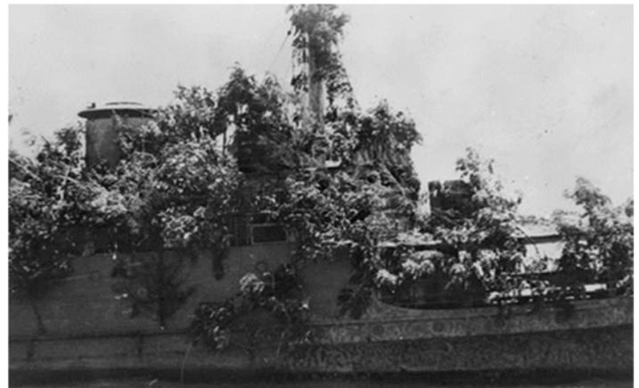
Close-up of the foliage used to camouflage the superstructure of the ship
